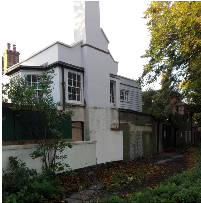
LOCATION A WITHOUT POLE
